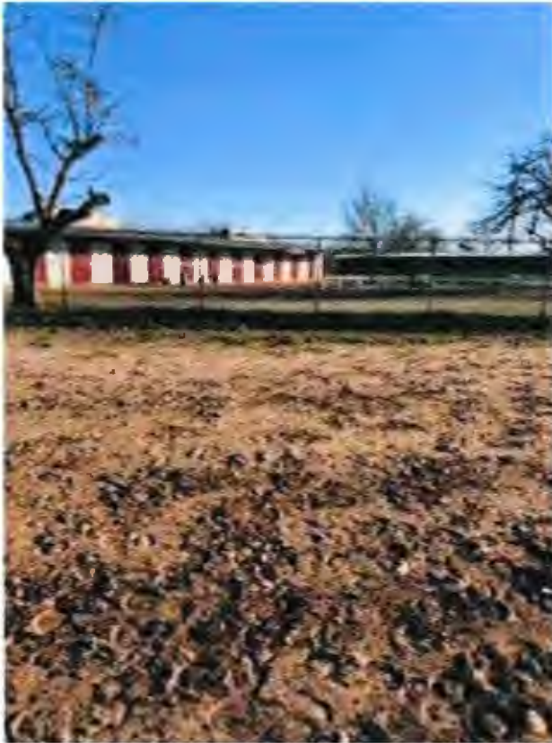
(View from racetrack, northeast corner – Barns D thru I)
