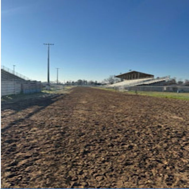
View from ¼ chute towards Finish Line
